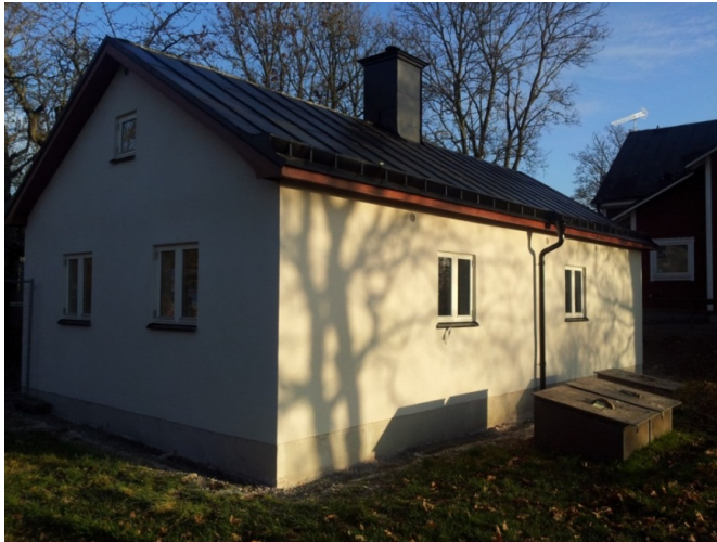
Skå skola Undercentral november 2013
